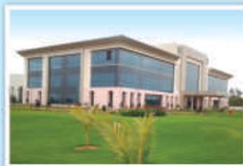
Vadodara Larsen & Toubro Limited Switchgear Training Centre Behind L&T Knowledge City, Near Village Ankhola, Vadodara - 390 019. Tel: (0265) 245 7805 E-mail : STC-VADODARA@LNTEBG.COM
