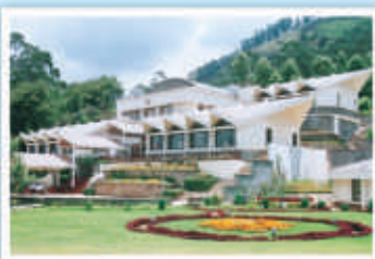
Coonoor Larsen & Toubro Limited Switchgear Training Centre Ooty-Coonoor Main Road, Yellanahalli P.O., The Nilgiris - 643 243. Tel: (0423) 251 7107 Fax: (0423) 251 7158 E-mail : STC-COONOOR@LNTEBG.COM
