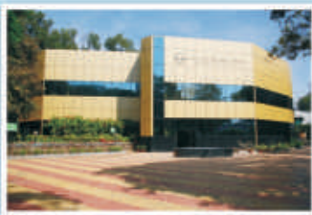
Pune Larsen & Toubro Limited Switchgear Training Centre T-156/157, MIDC, Bhosari, Pune - 411 026. Tel: (020) 2712 0037 / 2712 0653 Fax: (020) 2712 2933 E-mail : STC-PUNE@LNTEBG.COM
