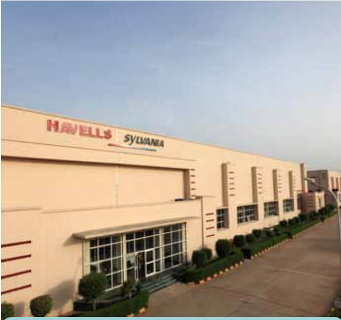
Neemrana Lighting Plant
